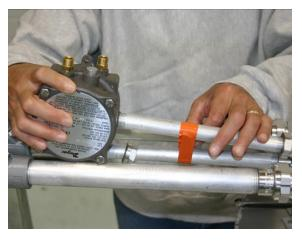
Carefully swing the switch 180° so it is out of the way and rests on top of the conduit connected to the control box. Use electrical tape to secure.
