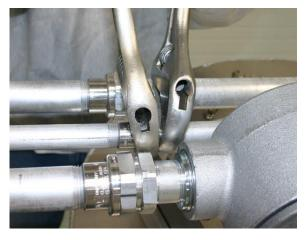
Use two large adjustable wrenches to loosen the ½" electrical union on the pressure switch conduit.
