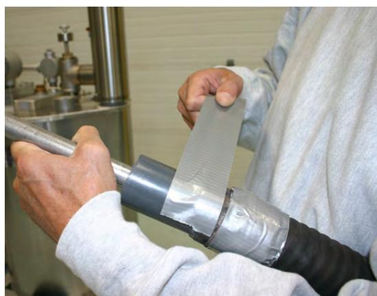
Prepare a shop vacuum with 48” piece of 3/4” tubing. Use 3/4” Electrical Metallic Tubing (EMT). Duct tape the tubing to the end of the vacuum hose.
