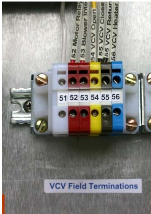
Figure 4 – FALCO Control Box Terminations
