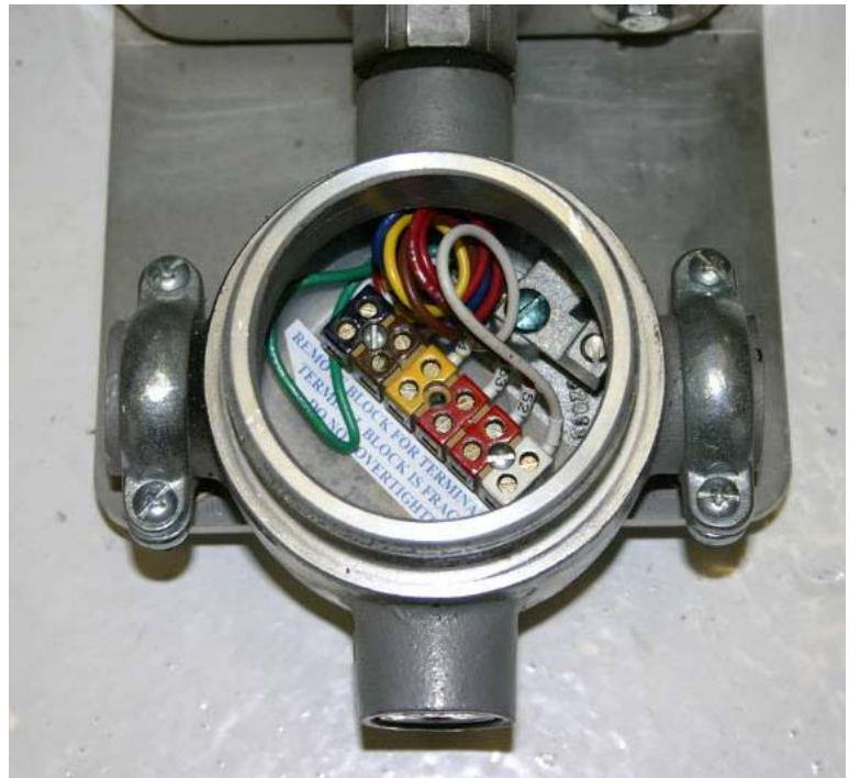
Figure 5 - VCV Conduit Body Terminations
